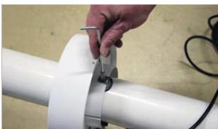
Clamp the unit with the bolts with hexagon tool nr. 4
