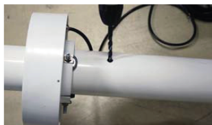
Drill a 11 mm hole under the unit
