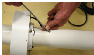
Use a cable spring to pull the cable through the pole
