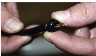
Place the tulle over the cable
